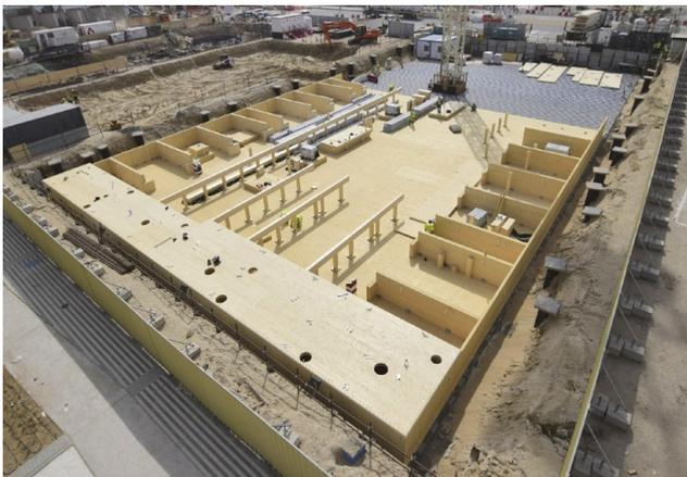
Figure 3: Timber foundation
